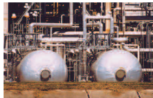
Fractional distillation column ( above ) is the most characteristic feature of a refinery. The catwalks at various levels provide access for maintenance. The column is at the Premcor refinery in Port Arthur, Texas. Insulated, bullet-tank reactors ( below ) are at the ExxonMobil refinery in Chalmette, Louisiana.
