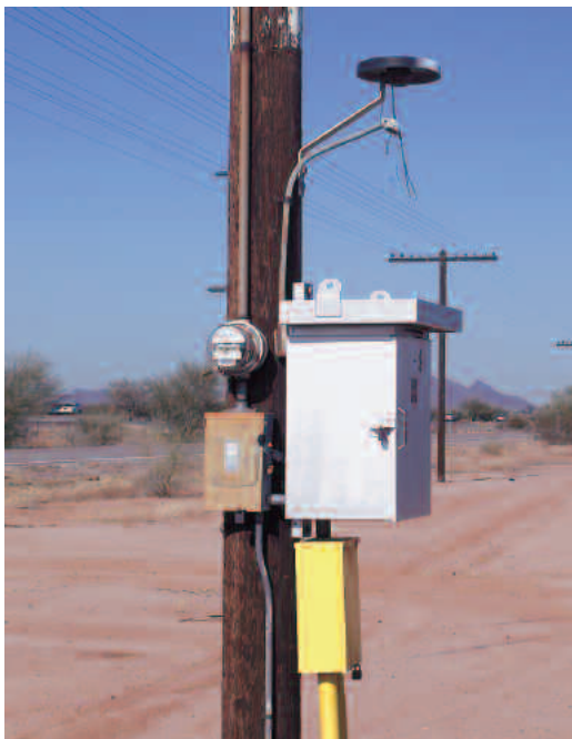
An anticorrosion device along the route of a petroleum pipeline in southern Arizona generates a small voltage opposing natural electric currents that would eat away the metal of the pipe. The circuitry for the protective device is inside the metal box; the black-and-white disk above the box spins when the current is flowing, as an indicator that the system is working.
