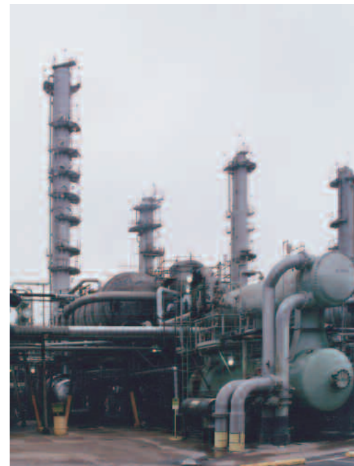
An alkylation plant at Pascagoula ( above ) also relies on bullet-tank pressure vessels, but in this case they are laid down horizontally; one large tank is visible here behind the smaller drums of a heat exchanger. The unit also includes several tall distillation towers.
