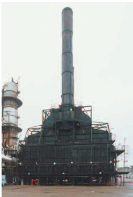
A feed heater at the ChevronTexaco refinery in Pascagoula, Mississippi, heats crude oil to about 700 degrees Fahrenheit. There are gas burners near the bottom of the unit; tubes lining the walls carry the feedstock to the heater. This furnace and another just like it at Pascagoula process 325,000 barrels of oil per day.
