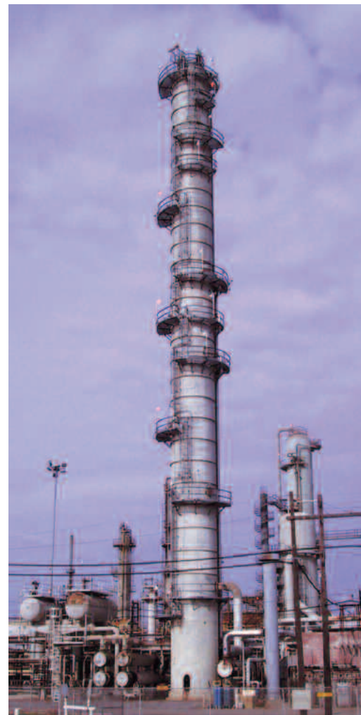
Fractional distillation column ( above ) is the most characteristic feature of a refinery. The catwalks at various levels provide access for maintenance. The column is at the Premcor refinery in Port Arthur, Texas. Insulated, bullet-tank reactors ( below ) are at the ExxonMobil refinery in Chalmette, Louisiana.
