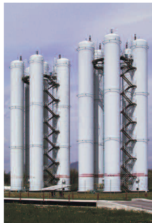
High-pressure cylinders store natural gas in a smaller volume than the low-pressure rigid and telescoping gasholders. The cylinders are in Ljubljana, Slovenia.
