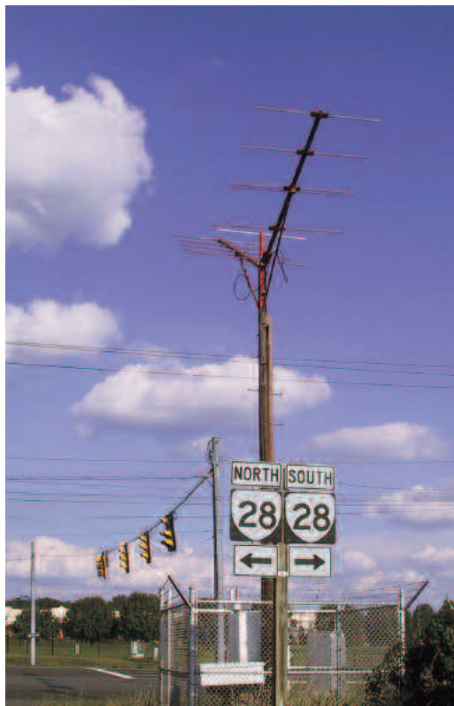
Marker beacons are another component of the instrument landing system, which tell the pilot how much distance remains to the runway threshold. Above is an outer marker, four miles away from the touchdown point, on one of the approach paths to Dulles airport in Virginia. Below is a middle marker, 3,000 feet out from the threshold.
