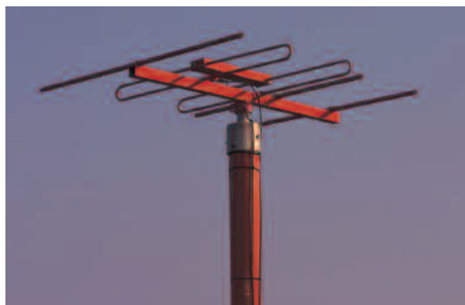
Marker beacons are another component of the instrument landing system, which tell the pilot how much distance remains to the runway threshold. Above is an outer marker, four miles away from the touchdown point, on one of the approach paths to Dulles airport in Virginia. Below is a middle marker, 3,000 feet out from the threshold.
