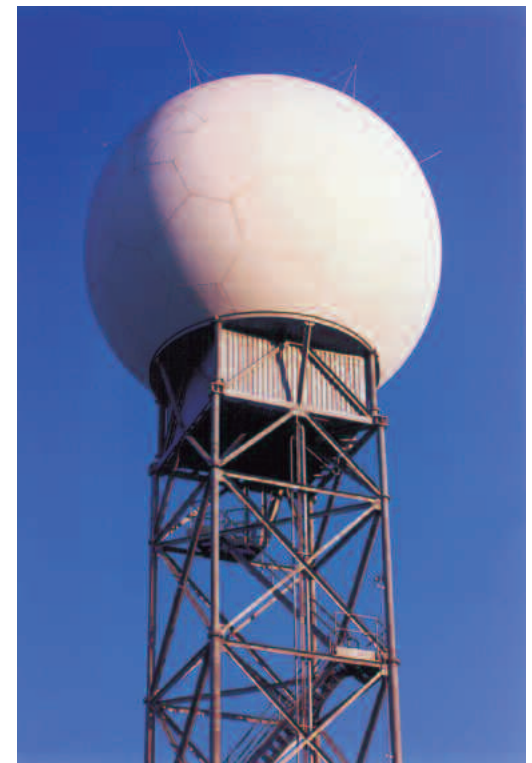
Radomes like this one in Pennsauken, New Jersey, also house antennas for weather radar.
